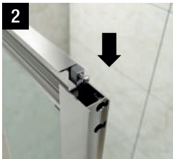
Slot the horizontal profile and screws into upright using guide channel until flush.
