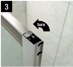
Secure screws into position using dedicated access holes.
